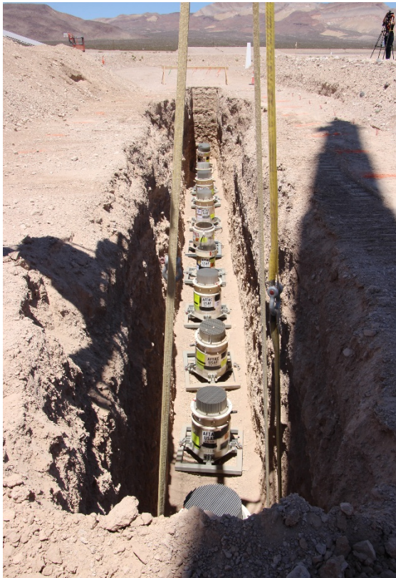
Fig. 3 RTGs Disposal at the NNSS
